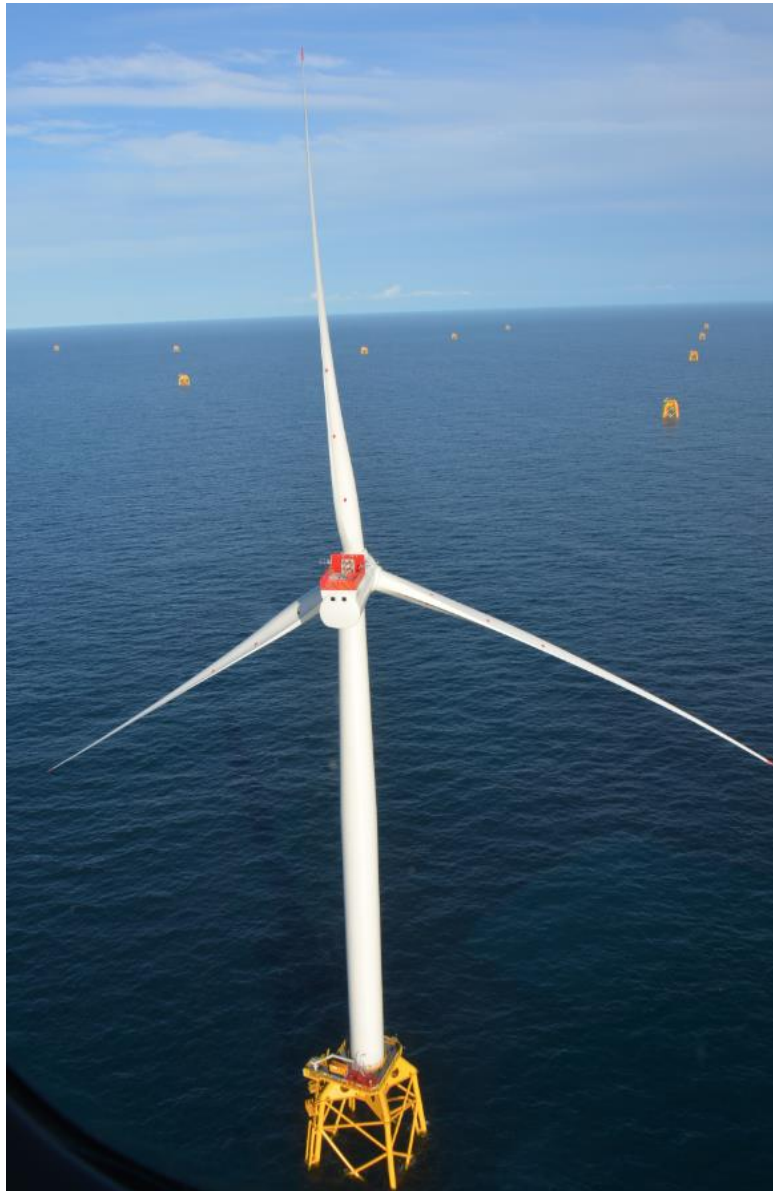
Fig. 5 Siemens SWT-7.0-154 WTG installed at Beatrice OWF
