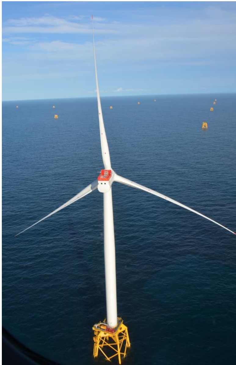
Fig. 5 Siemens SWT-7.0-154 WTG installed at Beatrice OWF
